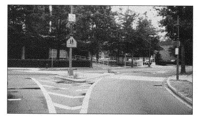
FIGURE 11–6. Factors such as sight distance, crash history, vehicular speeds, age of children, and other locational characteristics should be considered in selecting traffic control devices at school crossings.
