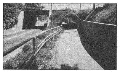
FIGURE 10–3. Pedestrian tunnels or underpasses generally involve ramps below ground, or at the grade of another roadway.
