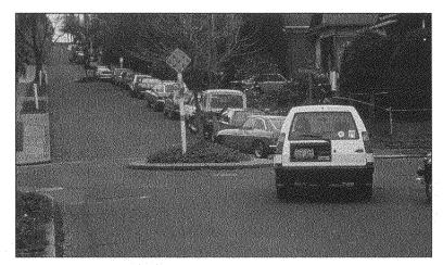
FIGURE 12–4. Traffic circles (minicircles) separate points of conflict within an intersection and often slow speeds of vehicular traffic.
