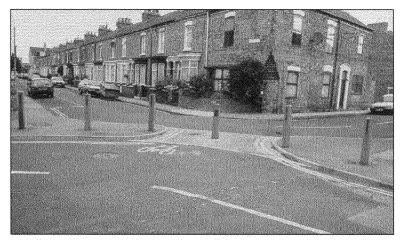
FIGURE 12–2. A diagonal diverter is a barrier placed diagonally across an intersection to convert it into two unconnected streets. This is an example from England, which allows free access to pedestrians and bicylists.
