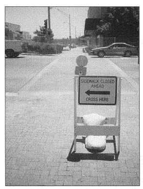
FIGURE 15–2. Ample advance notification of sidewalk closures is important.
