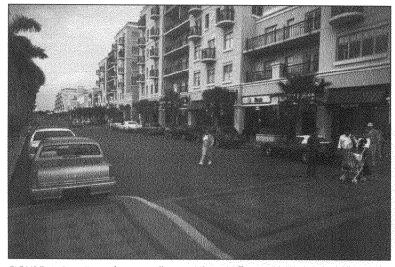
FIGURE 6–3. Raised crosswalks provide a traffic-calmed environment and elevate pedestrians to make them more visible to motorists.
