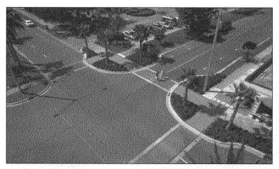
FIGURE 12–7. Streets narrowed at the crosswalk reduce the pedestrian exposure to vehicular traffic.
