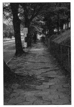
FIGURE 3–11. Poorly maintained sidewalks may result in trips and falls.
