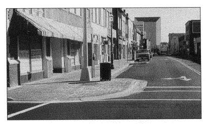
FIGURE 9–8. Chokers or bulbouts improve sight distance between motorists and pedestrians and shorten the crossing distance for pedestrians.
