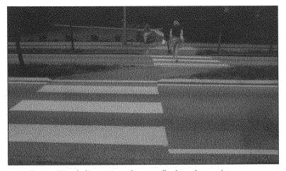
FIGURE 6–4. Angled or staggered crosswalks through a median can encourage pedestrians to cross one half of the street at a time.
