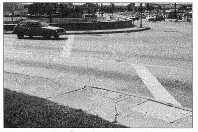
FIGURE 6–8. Angled or offset stop lines may help improve driver and pedestrian sight distance on some multi-lane approaches.
